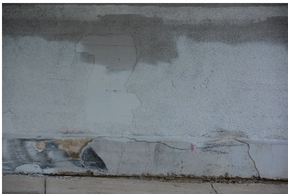
Figure 11: Typical condition issue with the cementitious coating, seen under the bridge on the north side.
