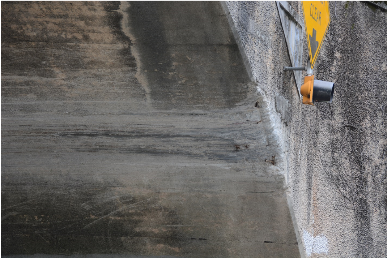
Figure 8: Detail of underside of bridge (barrel and arch ring) showing damage from vehicle impact.
