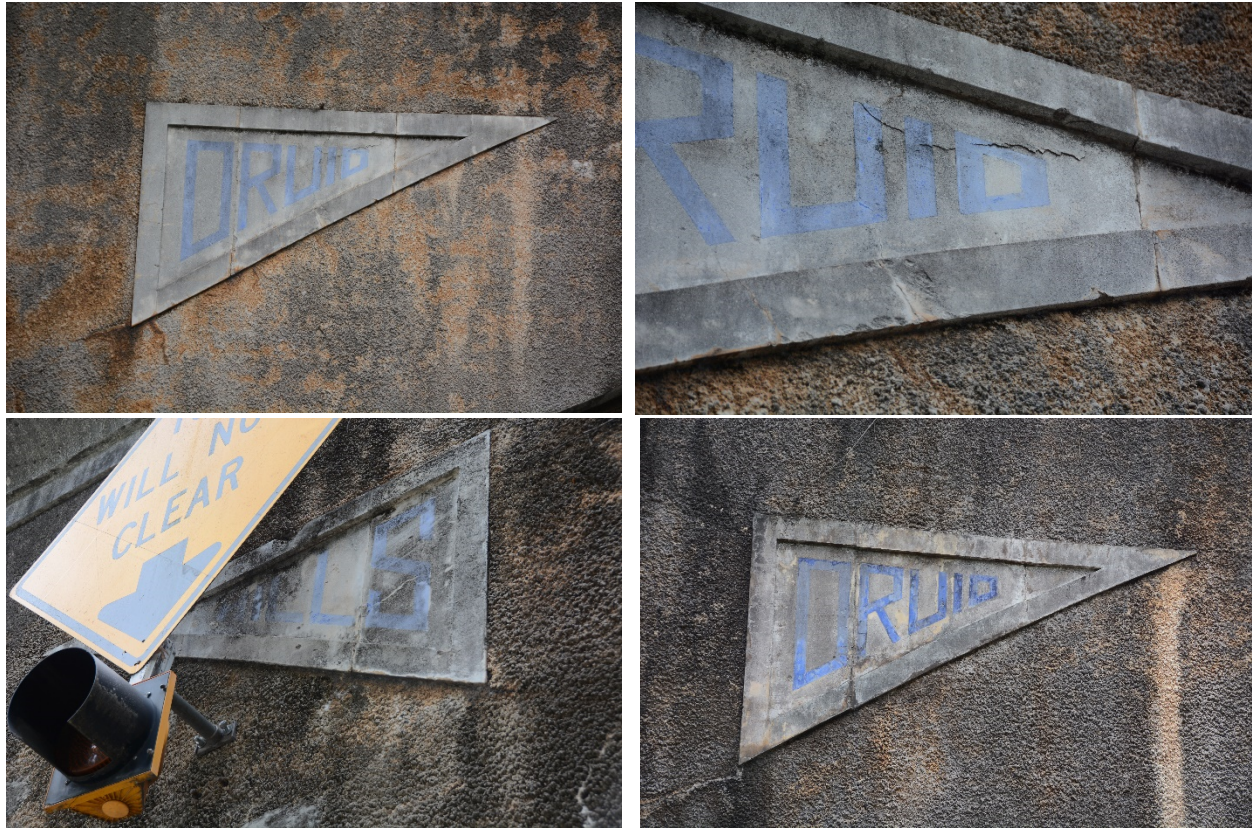
Figure 12: Details of triangular spandrel panels, clockwise from top-left: northwest spandrel panel, detail of area of potential spall on northwest panel, southeast panel, and northeast panel. Southwest panel is shown in Figure 9.
