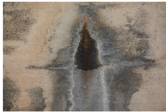
Figure 10: Detail of small fissure and active water seen under the bridge near apex of arch.
