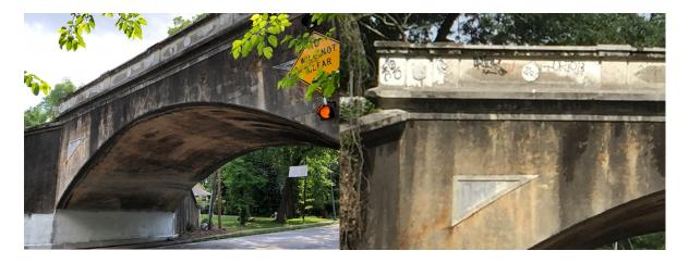
This photo shows the current dilapidated state of our bridge, an excellent example of the reinforced concrete arch bridge. As the report states, *The Druid Hills Railroad Bridge is a significant example of its type/design and is among the oldest extant reinforced-concrete bridges in the Georgia Historic Bridge Inventory. It is one of the few reinforced concrete arch bridges in the Inventory with decorative detailing.*
